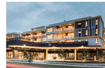
North Village, Kellyville – 209 Apartments + 2,760sqm Retail
