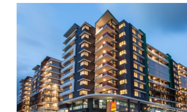
The Charles, Canterbury – 229 Apartments + Woolworths + 8 Shops
