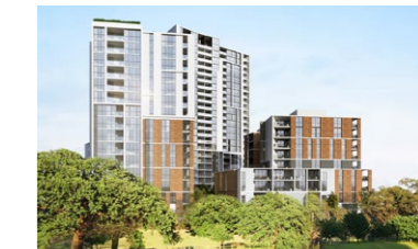
Highline, Westmead – 555 Apartments
